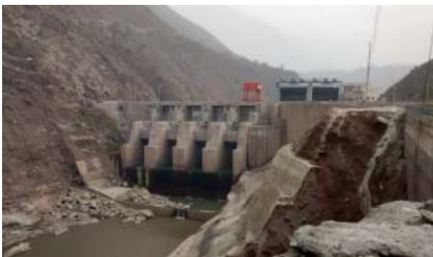
Accelerograph installed at Uri-II project, J&K
